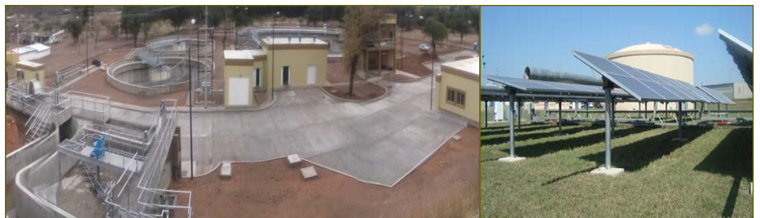
Los Alisos Wastewater Treatment and Conveyance Project and the on-site solar energy plant.
